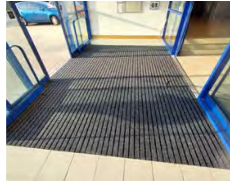
Surface mounted using KUB268 aluminium trim
